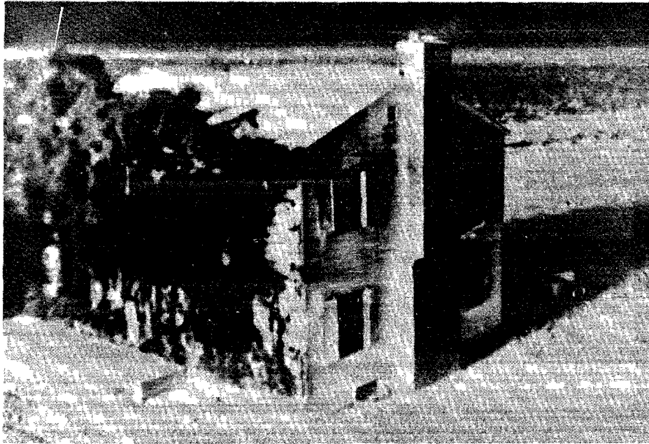
Fig. 7.1. Heat radiation charred the paint on this house, which had been painted white to reflect heat rays. The charring instantaneously produced the smoke. However, precautions had been taken to prevent this typical U.S. house from being destroyed by fire, because the test was made to enable engineers to study the effects of blast, rather than fire. The house was demolished by the 5-psi overpressure blast that struck seconds later, but it did not burn.
