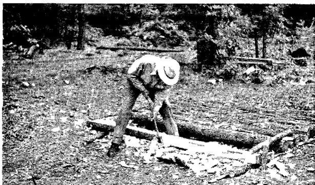
Fig. D.17. Hewing flat sides on a pole with a sharp ax.
