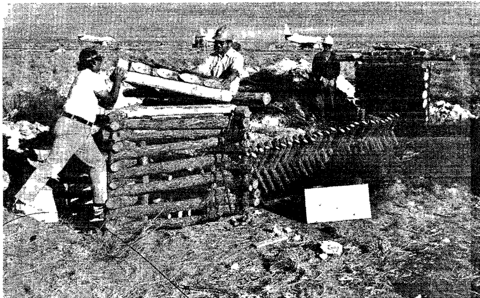
Fig. D.12. Completed frame of Chinese "Man" Shelter showing its two ORNL-designed entryways (one at each end) and triangular blast doors made of poles. Before covering the triangular vertical entries with earth, tree branches were placed vertically over the sides; the branches then were covered with bedsheets. Horizontal branches, also covered with bedsheets, were laid over the rest of the shelter frame. After being covered with earth, this shelter was subjected to 1-kiloton blast effects. Multiple earth arching over and around this yielding structure prevented both the small poles and the bedsheets from being damaged at 20 psi.
