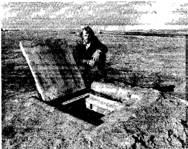
Fig. D.13. Blast door surrounded by 4 blast-protector logs that were notched and nailed together. The wet, mounded soil had been compacted by the blast but not blown away.
