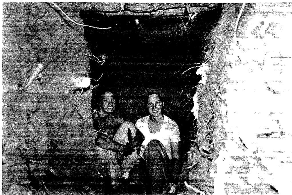
Fig. 5.2. Two non-athletic college girls who completed a 4-person Pole-Covered Trench Shelter in 35\frac{1}{2} hours, despite tree roots.
