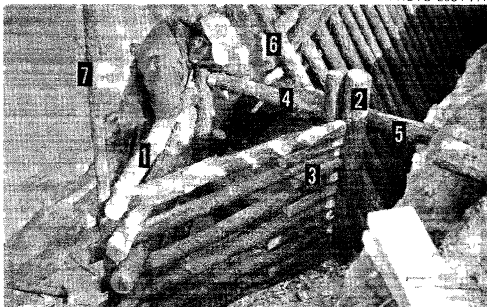
Fig. D.10. Uncompleted lower section of a vertical triangular entry.
