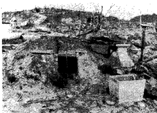
Fig. 1.5. Undamaged earth-covered family shelter in Nagasaki.
